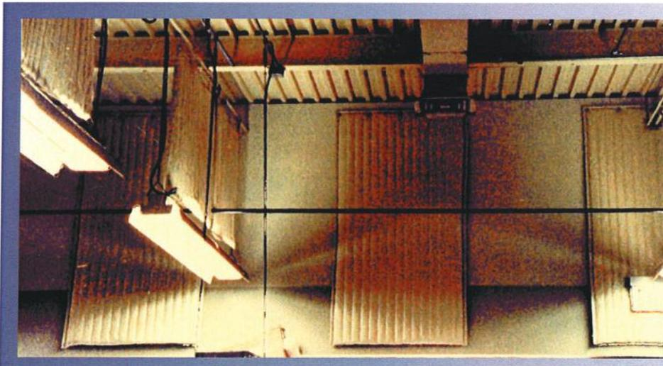
*Clearer and easier communication was achieved in this manufacturing plant with QFA-10 Overhead Sound Absorption Baffles and Sound Absorption Wall Panels-shown with optional straight stitch pattern and tan-colored vinyl facing.*
